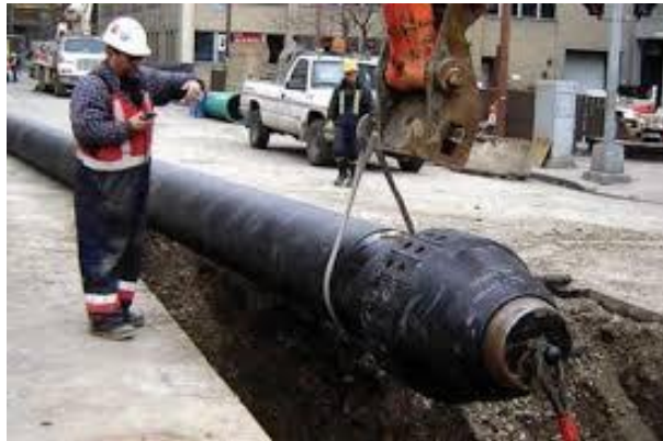
HDPE Burst Head
