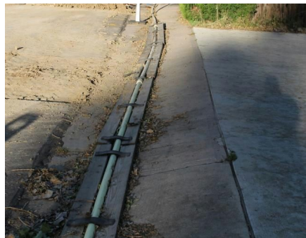
Figure 21 – Driveway Crossing with 6x2 Planks Strapped to 2” Restrained Joint PVC (Yellowmine)
