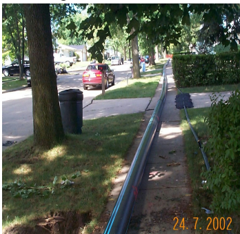
Figure 20 – Driveway Crossing w/ Cold Mix
