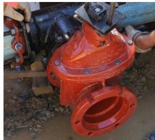
Figure 11 - Mechanical Joint Fittings & Restrainer Glands
